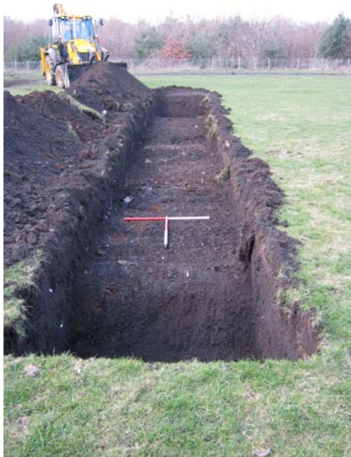
Fig. 7 - General view of Tr 11
