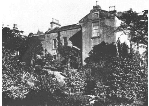
After Neill's death, Canonmills Cottage (pictured above) was occupied by descendants of his business successor William Fraser until 1898, when the company built a factory on the site. But it seems from a change in shape and orientation on maps that the original Cottage may have been substantially altered in 1859–60, when it was renamed in the P.O. Directory as Canonmills Lodge.
