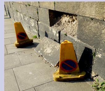
The seeming massive blocks lining the **embankment on Bellevue** are not as massive as first imagined, and some of the **facing stones** are now parting company from the **crumbly sandstone behind**. CEC is aware.
