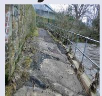
Heavy rain and localised floods scoured out sections of the Water of Leith Path between Newhaven Rd and Anderson PI just before New Year. Until fixed, this part needs extra care in poor light, post-refreshment, when walking without common sense.
