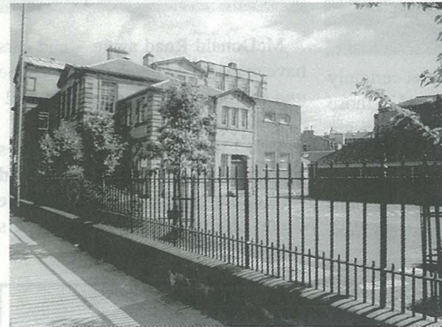
St. Mary's School in East London Street
