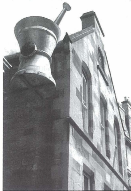
The Stafford Centre, 103 Broughton Street
