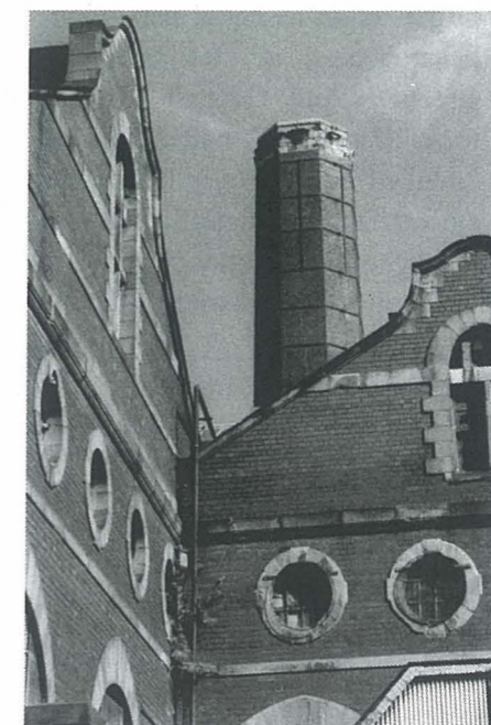
Some of the old bus depot buildings, seen from the rear of the site
