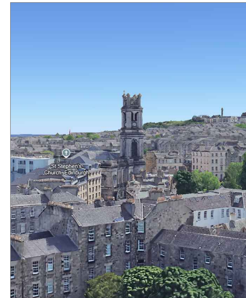
West Elevation (panels not visible)
