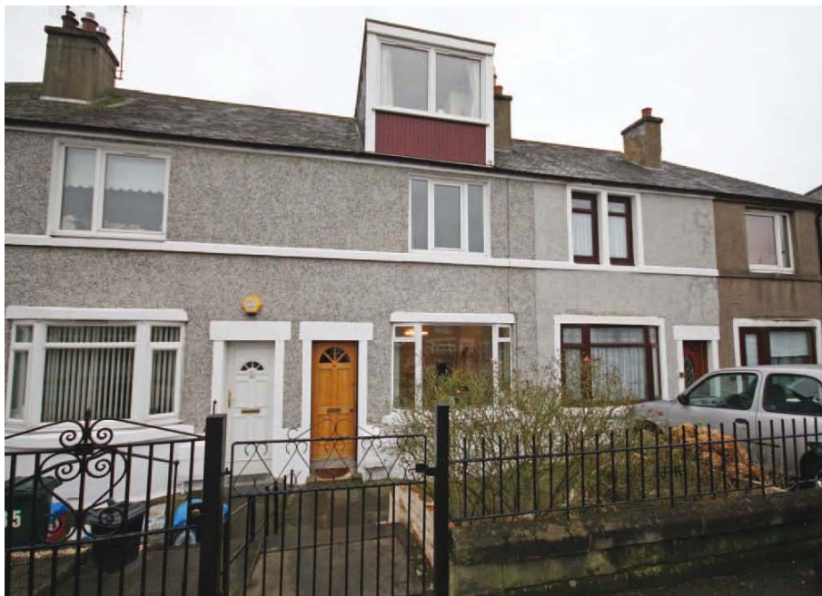
Image 4: Street view of 87 Annadale Street indicating shed dormer. 91 Annadale Street is at the extreme right hand of the photo. The black painted, continuous eaves gutter and associated fascia board are clearly evident.
