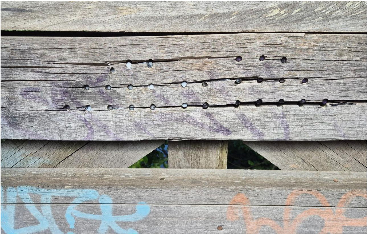
Figure 2: Top chord node – internal view.
