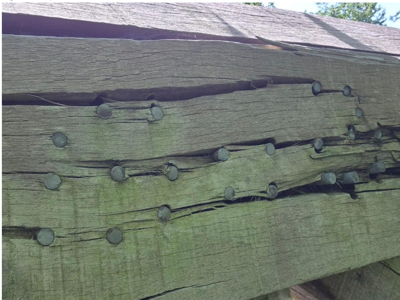
Figure 3: Top chord node – external view
