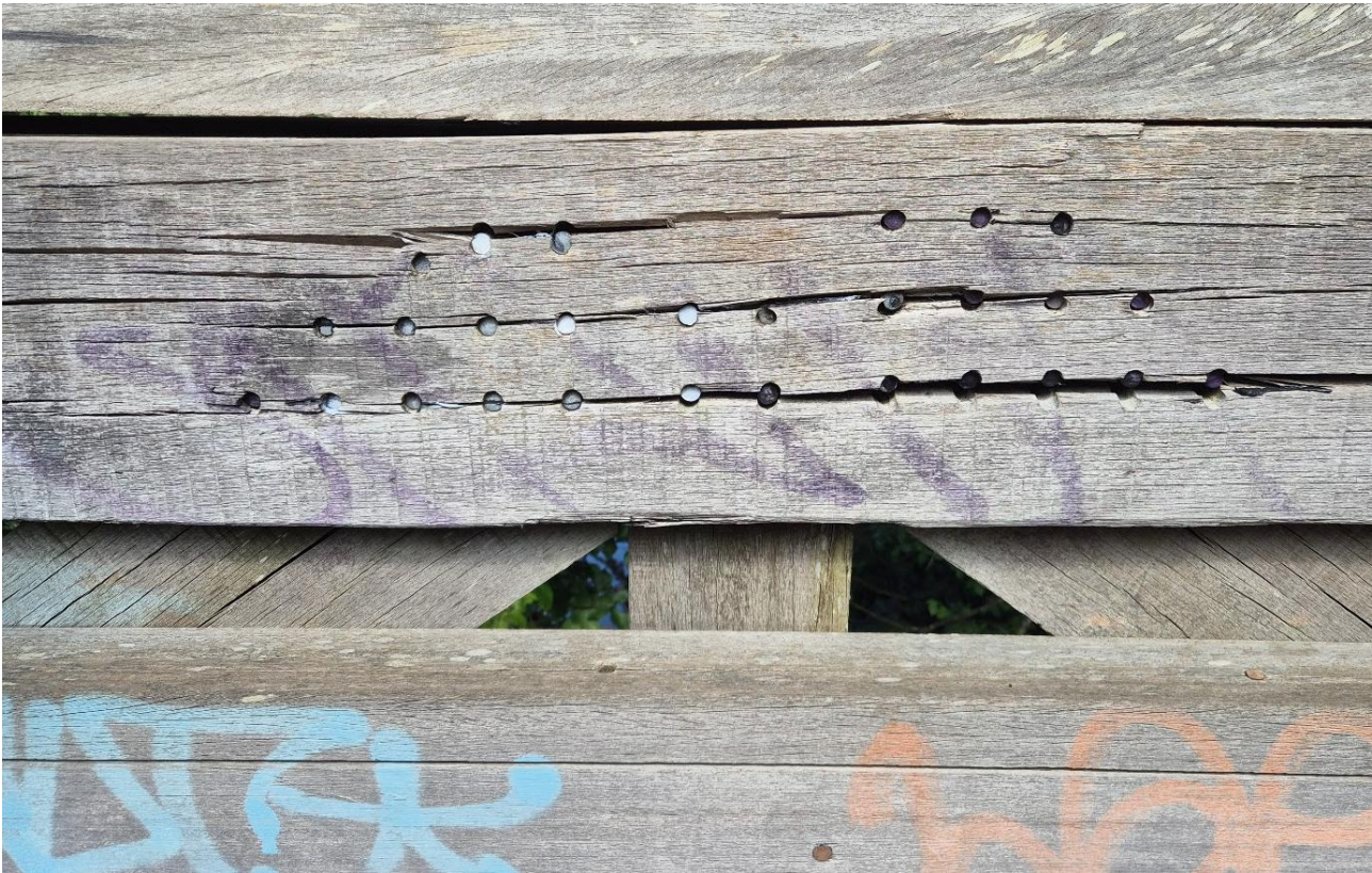
Figure 2: Top chord node – internal view.
